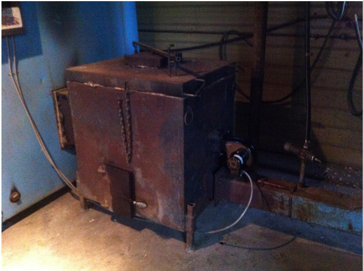
Figure 16: Waugh on-farm wood chip burner
